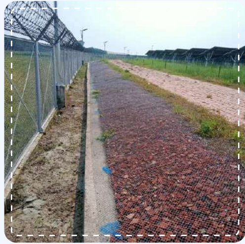
Slope Protection and HBB road
