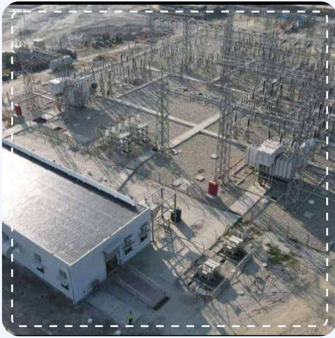
132kv/33kv AIS Substation
