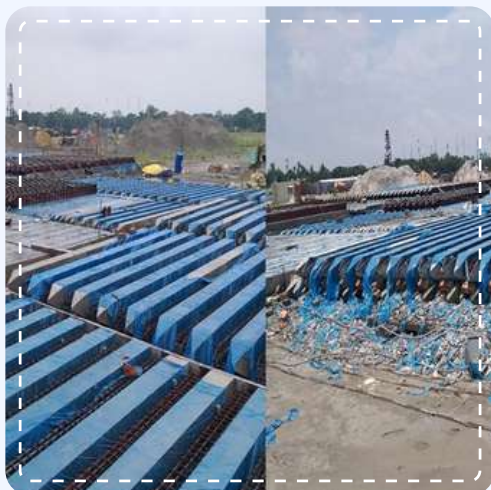
35MW Power plant precast pile manikganj (Spectra project)
